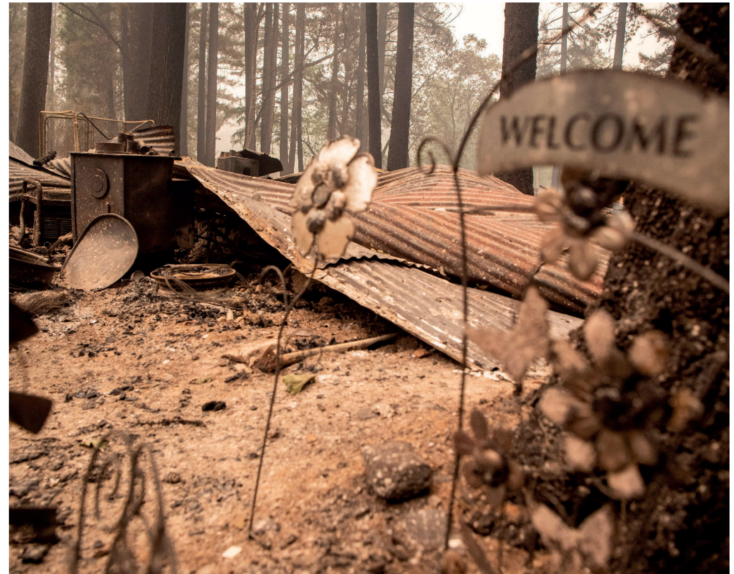
A HOME DESTROYED BY THE 2021 DIXIE FIRE IN CALIFORNIA.
